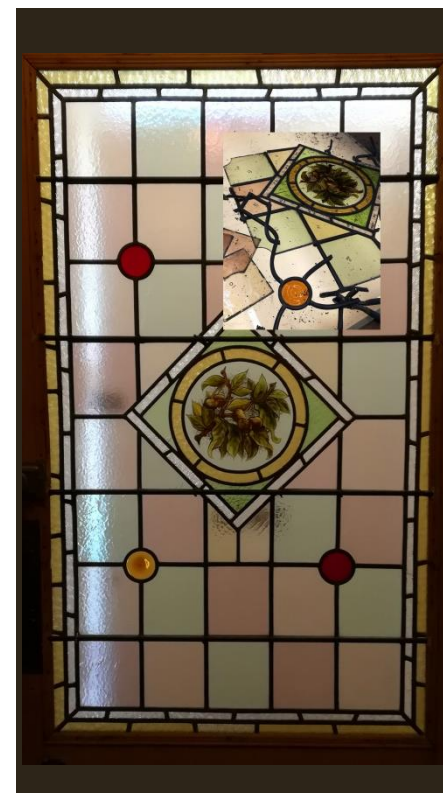
Restoration front door Dalziel PI
